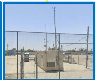
Compton Air Monitoring Station (SLA)
