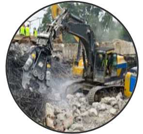
Construction or demolition sites
