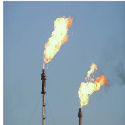
Figure 5b-2: A photograph of a flaring event at a refinery
