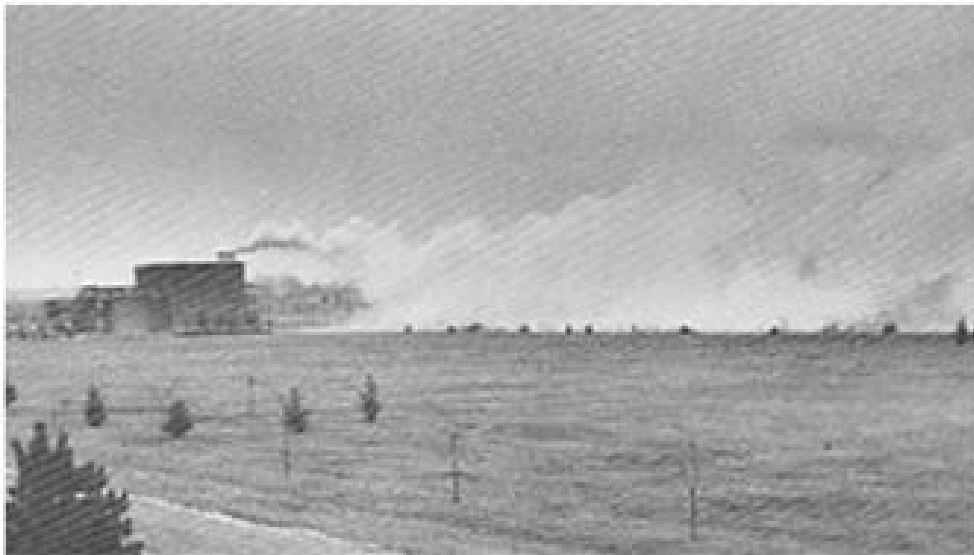
Figure 3-14 Downwash from a Short Stack – New Zealand Picture
